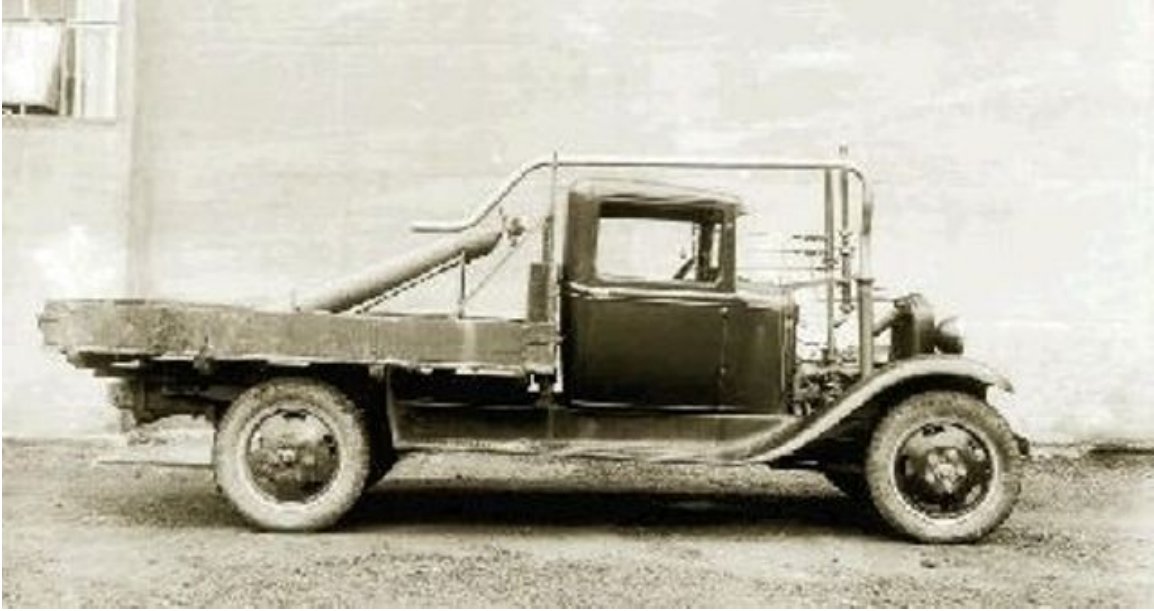
Pickup truck of the Norsk Hydro Company, converted to run on hydrogen gas. Illustration courtesy of the Oslo Technical Museum.
